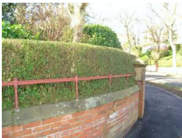
Image 6.3: Boundary wall with iron rail
